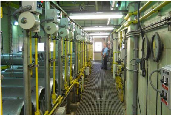
**P2-120N4 Actuators with custom built Local Control Stations for chlorine injection**
