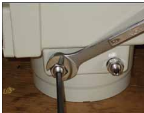
CCW Mechanical Stop
