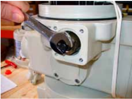
Loosen lock nut. Refer to step 5
