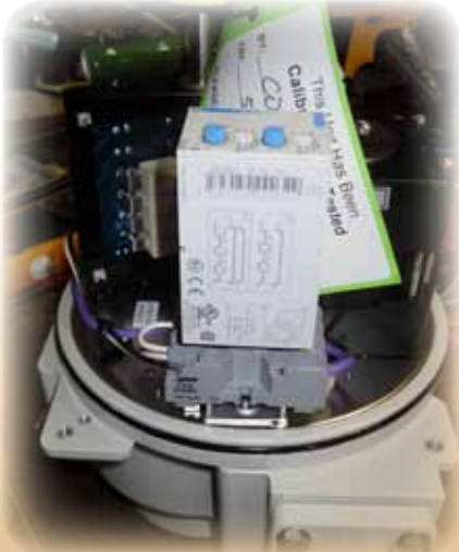
Timer Option installed in a P3-120VAC series actuator
